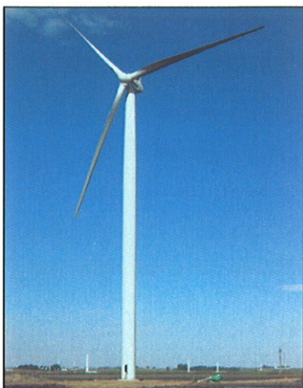
The blades on a wind turbine, such as this one in Iowa, are about 85 feet long.
