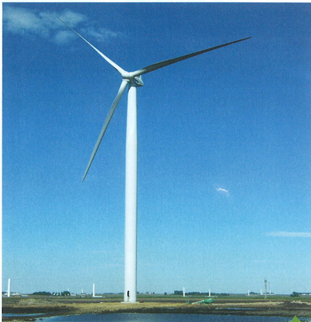
The first completed wind tower stands 262 feet. Each blade weighs 7.5 tons and is 131 feet long. Each massive foundation required 450 cubic yards of concrete weighing close to 1.5 million pounds.
